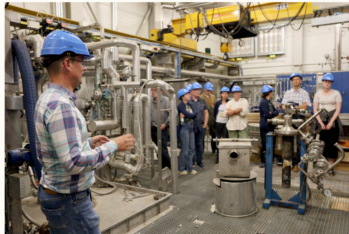
Fredrik Granberg, CEO at LTU Green Fuels, presents the pilot plant for the gasification of bioproducts to syngas and green fuels, at study visit in Piteå in 2024. Photo: Stina Johannesson.
